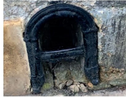
Dovers House, High Street, GL55 6HB
