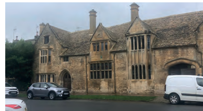
Figure 12: Grevel House; 14th Century, Grade I listed.
