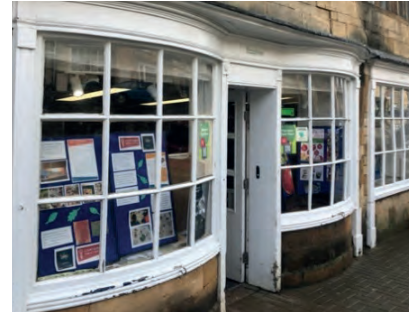
The Co-operative ("Co-op") 12-14 High Street, Chipping Campden, GL55 6HB
